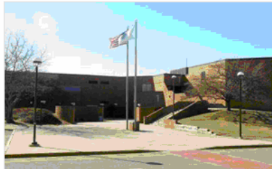
North Attleboro High School building.
